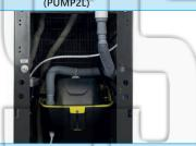
Pumps the water from the Drip Tray to Mains Drainage over a distance of 100m & a rise of 5m. Factory fitted only.
